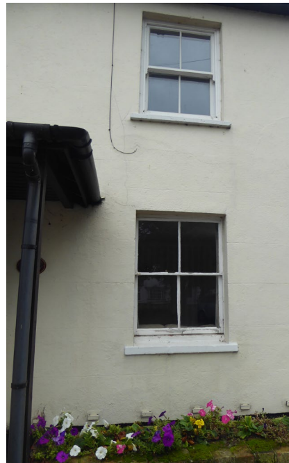
Figure 32 Traditional windows of Number 28 The Street
