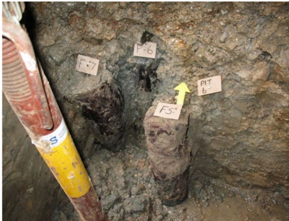
Figure 3 Three wooden piles beneath church tower.
