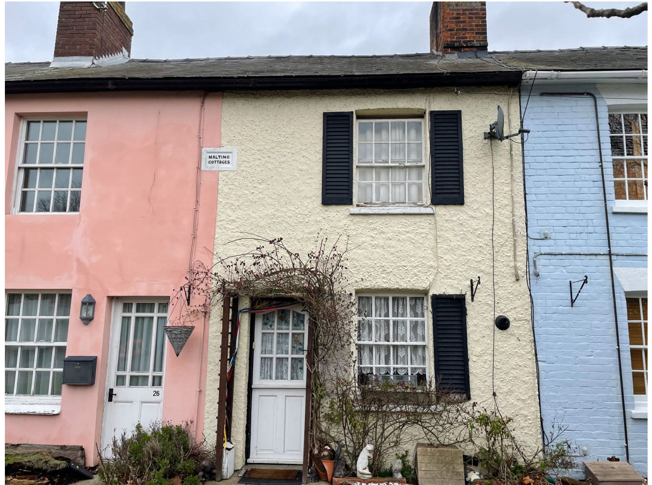
Figure 21 Close up of maltings Cottages
